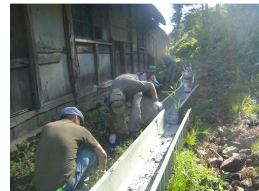
Maintenance of drainage ditch in the backyard
